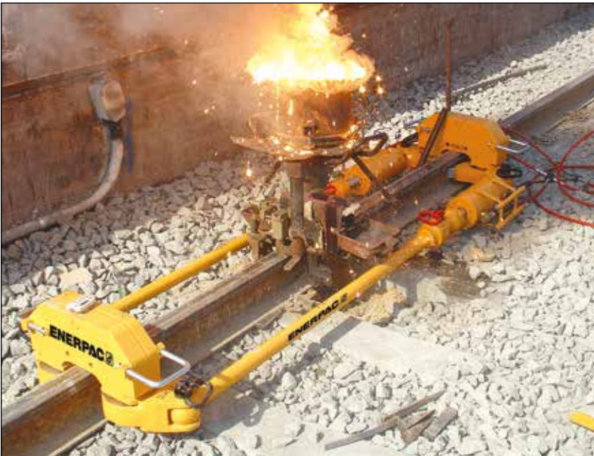
▼ Closure weld under neutral temperature using the RP-70 hydraulic Rail Puller
