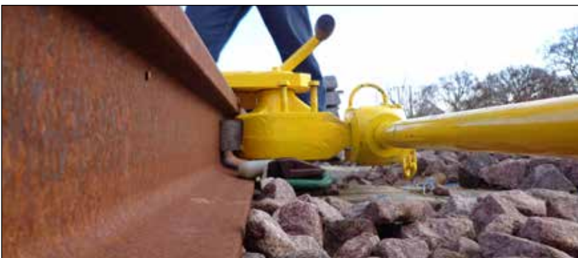
▼ RP70 Rail Puller in an obstructionless pull.
